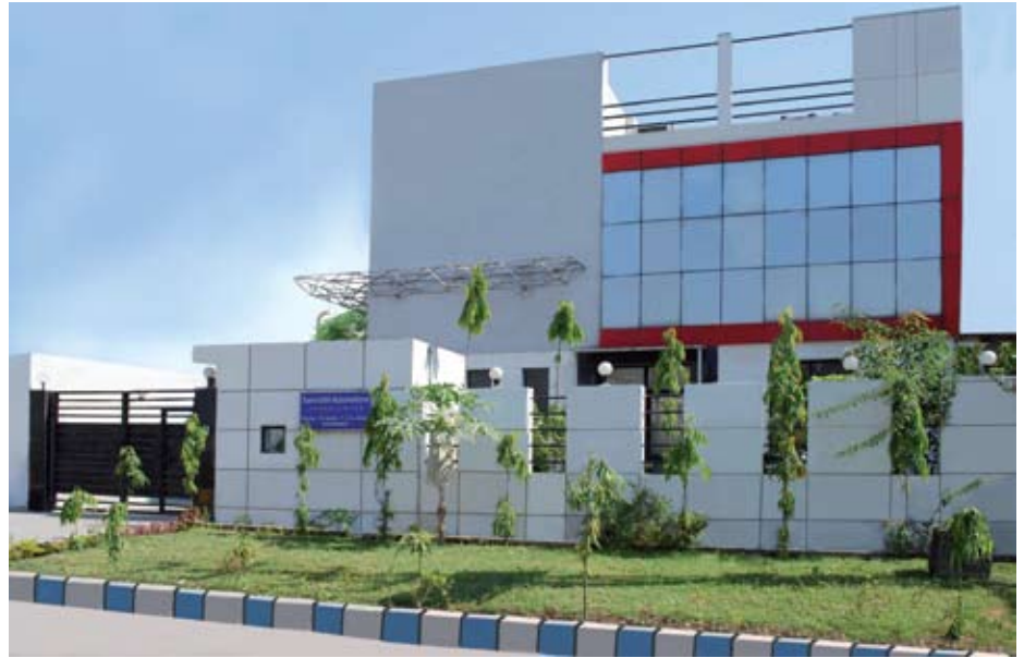
Sparsh Infrastructure – Manufacturing Facility at Haridwar
